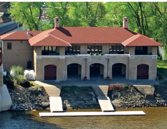
District heating service to the Minnesota Boat Club, located on Raspberry Island, will start in January 2008.
